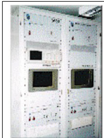
Surface Operations Cabin: Interior
